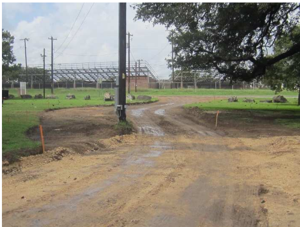
Lower Park Road realignment
